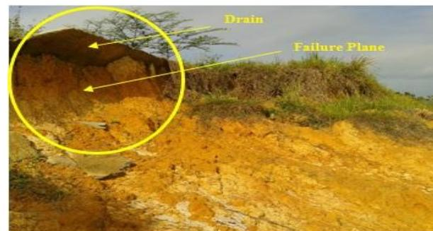
Fig. 3: Failure Plane beneath Slope Crest
